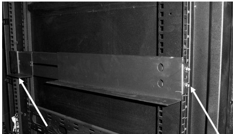
ASSEMBLE THE RAIL ONTO THE CABINET U-BAR WITH SCREWS AT FRONT & BACK USING MOVABLE NUTS
