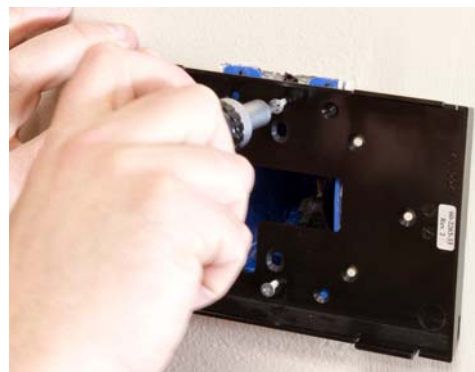
FIG. 5 INSTALLING THE BACK BOX TO THE GANG BOX.
